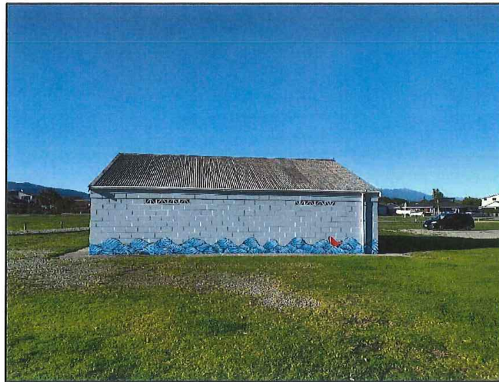
New murals at Carters Beach amenities block; note rusting roof
