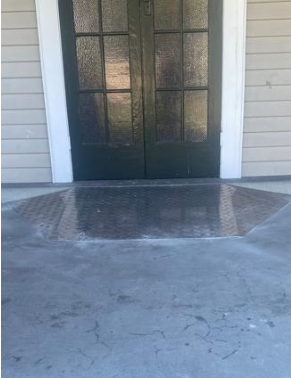
Ramp for womens refuge completed
