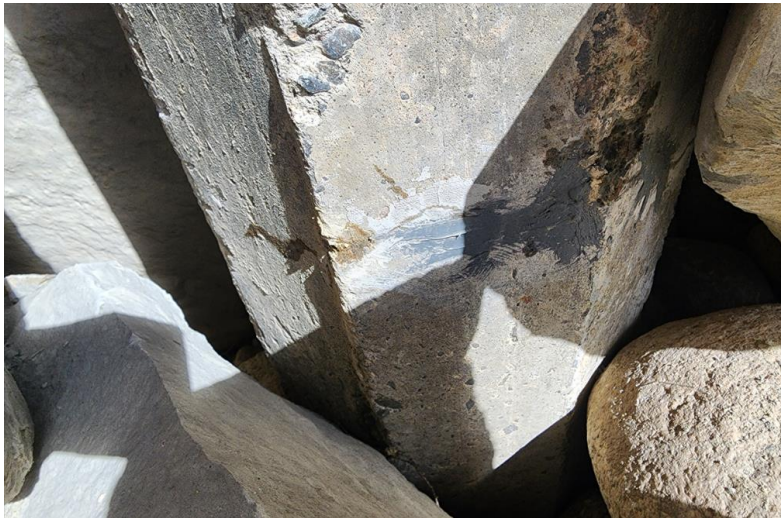
Rough Creek Bridge
