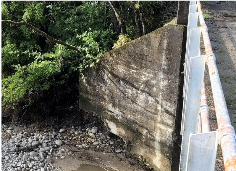
Gannons Creek Bridge
