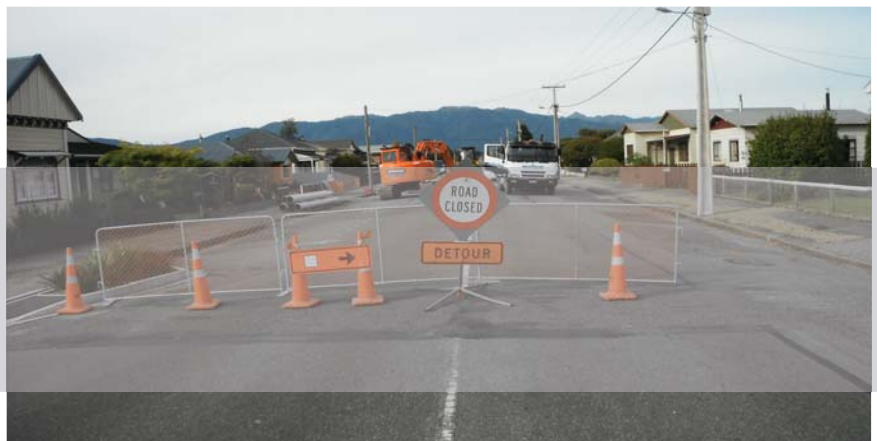
WestReef Services - Derby Street reconstruction, Westport
