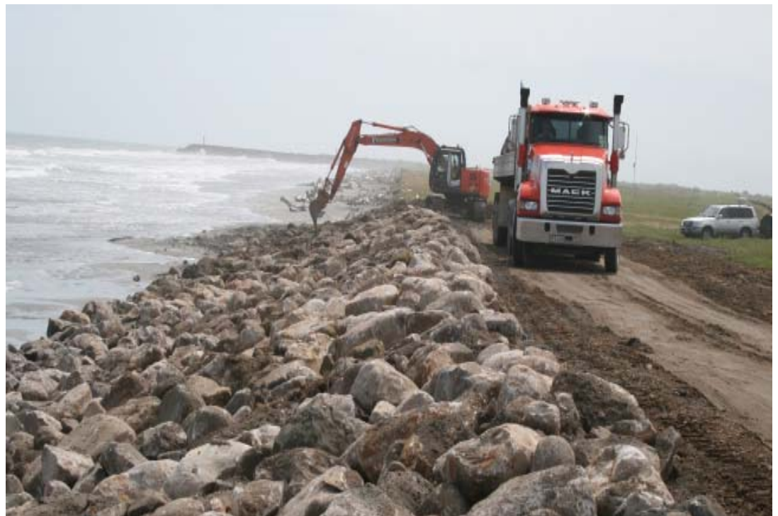
Rock Protection works - Westport Airport
